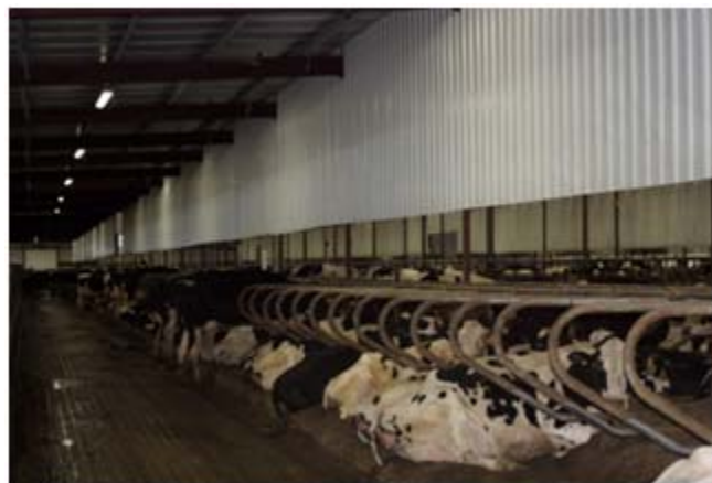
Picture 1. Metal baffles placed in between two rows of freestalls.
